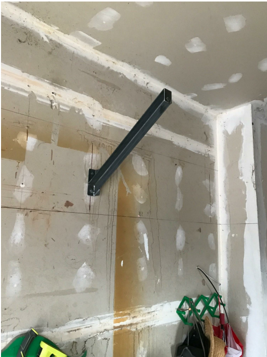
1. Horizontal and vertical layout. Lag first "Monster Bracket" to wall stud.
