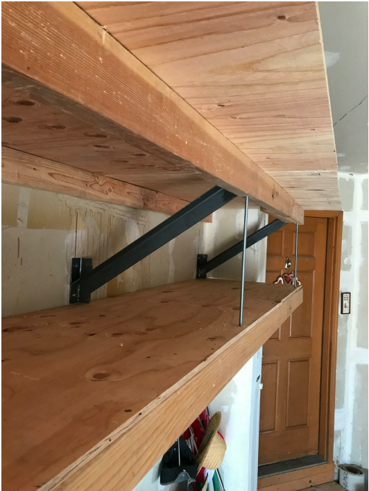
5. Install lower front ledger and shelf. In this application shown, the lower shelf is 18" tall (the minimum) and 24" deep. The upper shelf is 32" deep.
