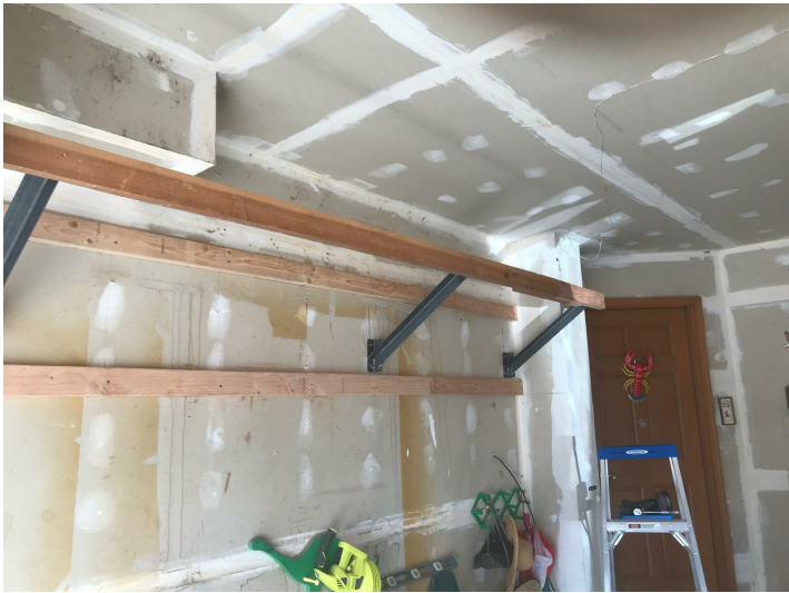
3. 18" tall shelving shown. Install upper front ledger.
