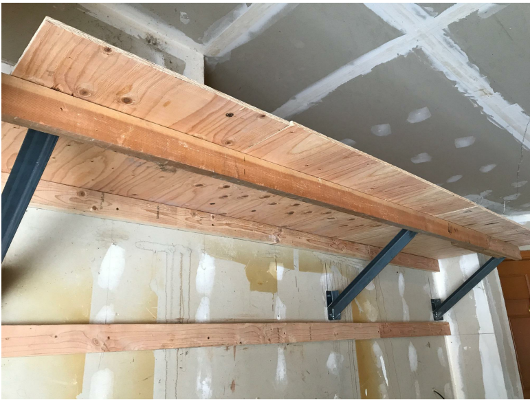
1. Prior to installation of threaded rod and lower front ledger and shelf.
