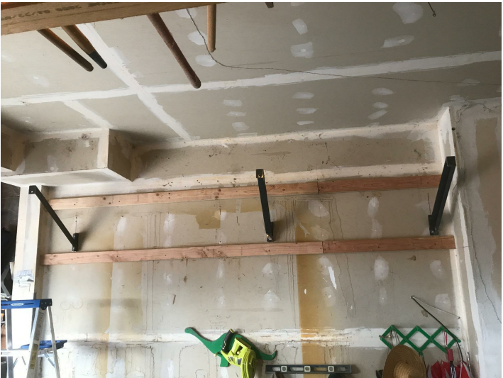
2. Two levels of shelving shown. Lag rear ledgers to wall studs. Install remaining "Monster Brackets" for the upper level shelving.
