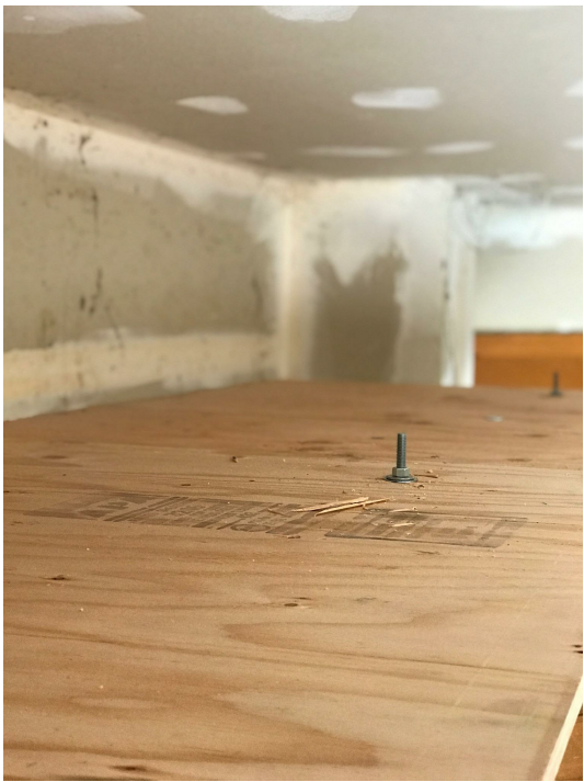
3. Top of threaded rod above upper front ledger and shelf
