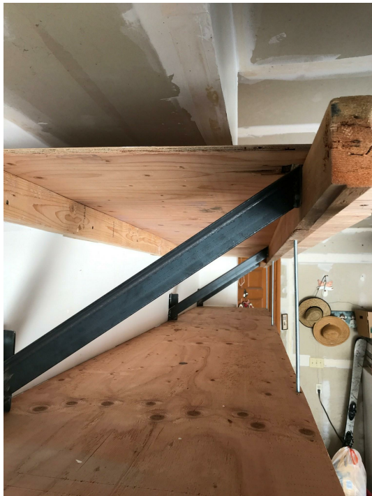
2. Section looking into garage. (32" top shelf, 24" second shelf x 18" tall)
