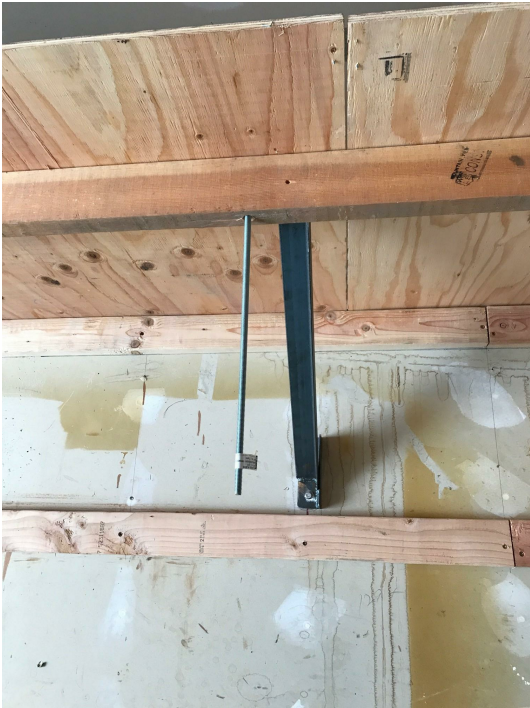
4. 32" deep upper shelf with 18" tall lower shelf shown. Install threaded rod.
