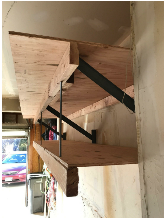
1. Section looking out of garage. (32" top shelf, 24" second shelf x 18" tall)
