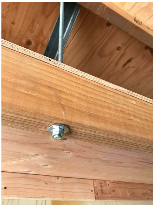
4. Bottom of threaded rod below lower front ledger and shelf
